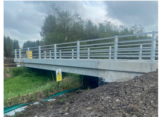
Figure 2: New bridge structure
